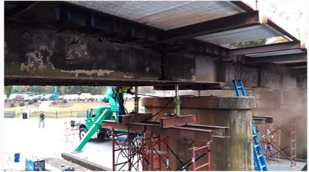
Raising the 11ft-8in "Can Opener" Bridge in Durham, NC
