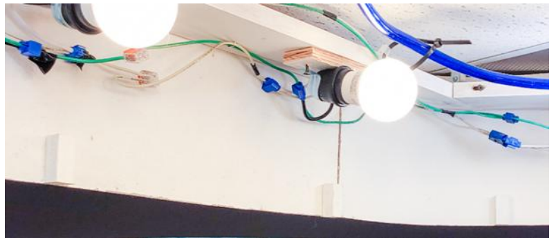
Photo 6 – Lights showing the suitcase connectors and inside of valance. Note the blocks of wood at the bottom of the valance used to attach the lighting louver which will hide the lights. The blue light rope is installed to simulate night.
