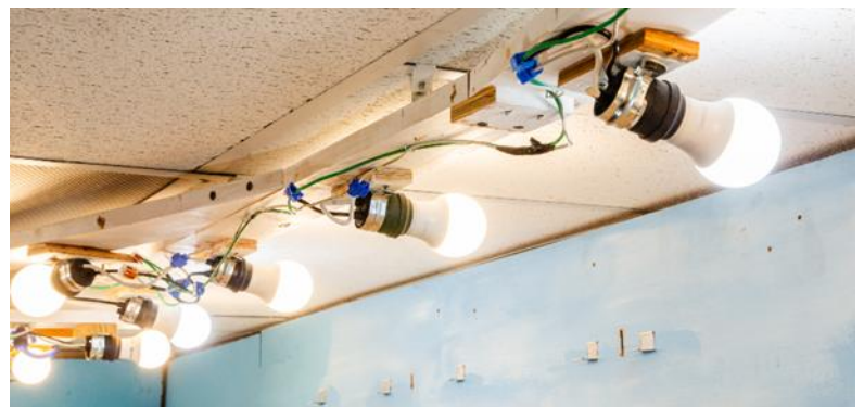
Photo 4 – Lights and board attached to the ceiling. Note the angle molding pieces on the backdrop to hold up the louver panels at the bottom of the photo. The slots in the backdrop support the cross tees.
