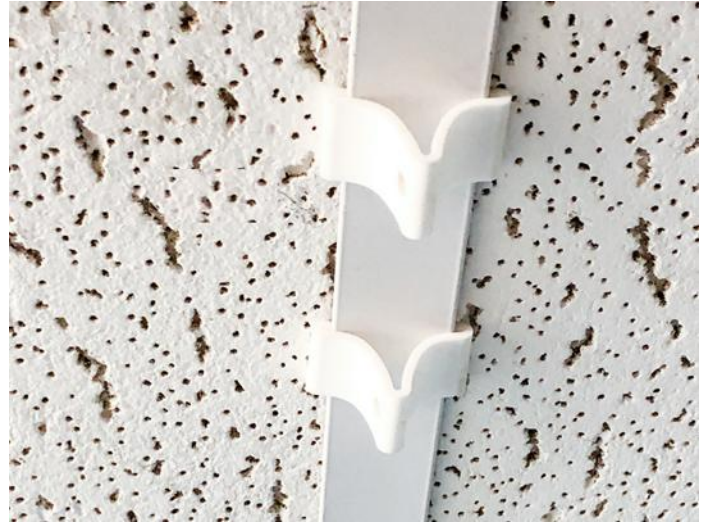
Photo 2 – Spread the clips so they fit over the cross tee. Make sure the clips are seated on the tee properly.
