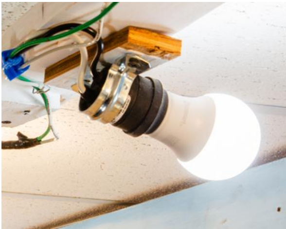
Photo 5 – Socket attached to board using 1" conduit strap with a 1/2" plywood spacer.
