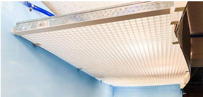
Photo 7 – Louver panel attached to backdrop and valance. The cross tee is needed to prevent the louver from sagging.
