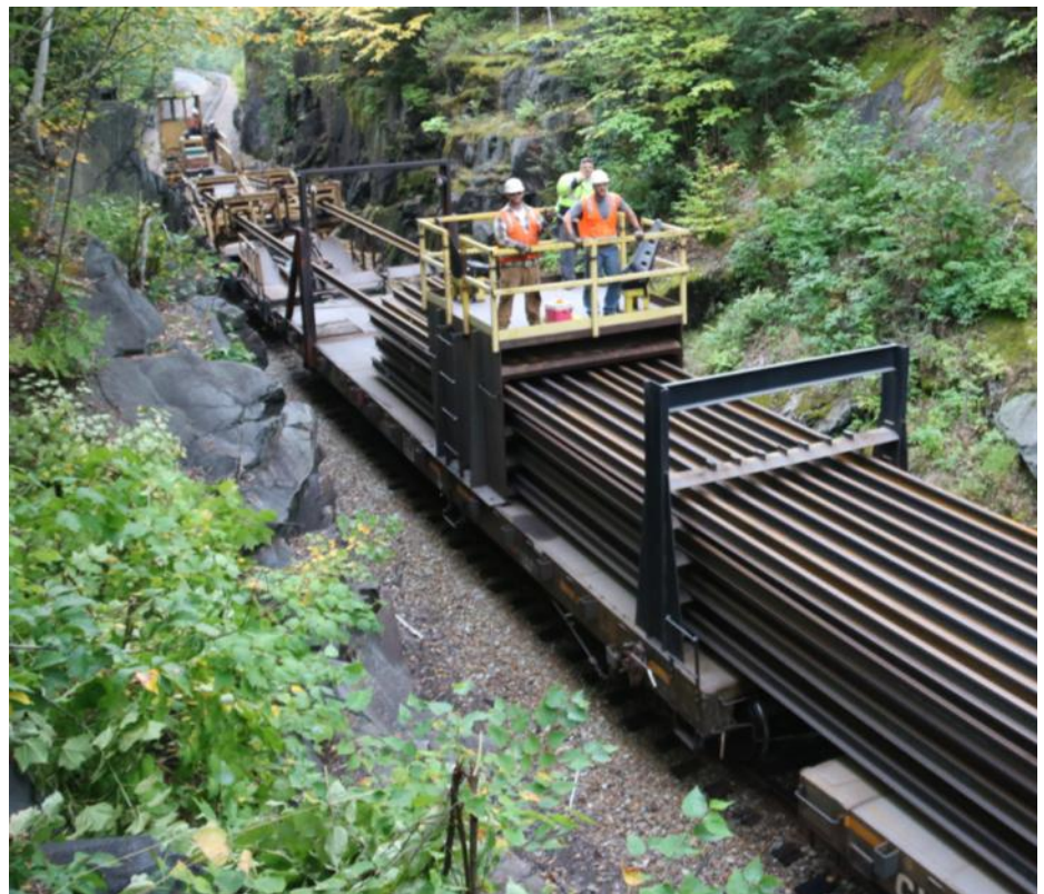
Rail Train on the Central Maine and Quebec near Onawa Road. At the rear of the train are the conductor and two crew who feed rail sections into the distributing equipment.. Photo by Harry Gordon
