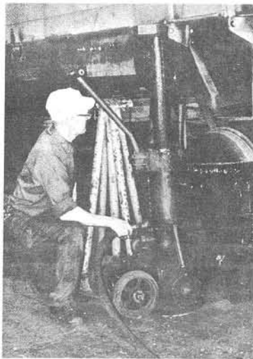
Waterville Shops employee Ralph Roberts preparing a boxcar for installation of trucks which have been modified with new roller-bearings wheel assemblies.
