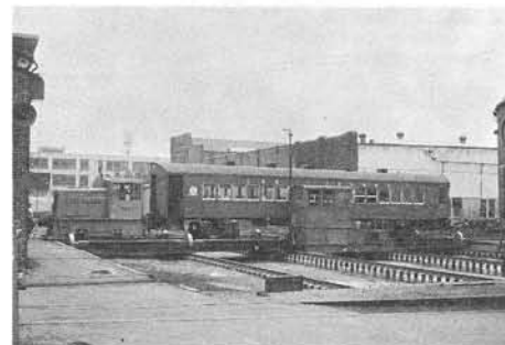
(Rothberg Photo) TRANSFER TABLE AT LIRR'S MORRIS PARK SHOPS WILL BE A FEATURE OF FALL PANTRIP
