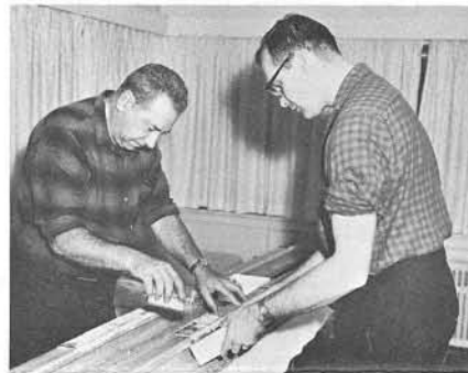
MAURICE BLEAU & JIM THOMPSON LAYING TIES & BALLAST. NOTE MATCHING ENDS OF INDIVIDUAL SECTIONS ARE DONE WHERE THEY MEET FIRST TO MAKE A PERFECT MATCH.
