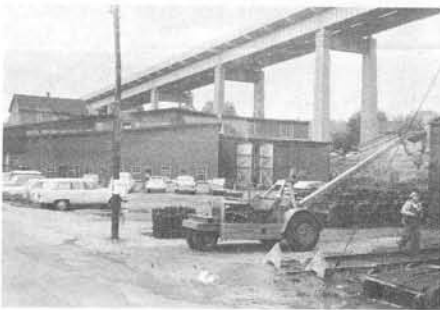
THE CENTRAL VERMONT'S 4-STALL ENGINE HOUSE AND TURNABLE IS JUST ONE OF THE MANY PROTOTYPE INSTALLATIONS TO BE SEEN IN THE NEW LONDON AREA.
