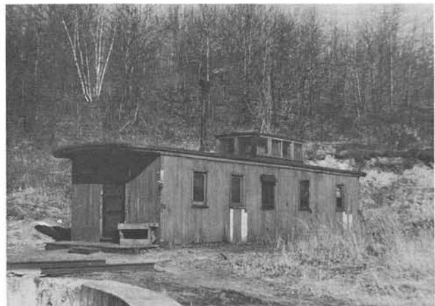
Here is a use for that old caboose which you were going to throw away. This one was the Boston & Maine bunk room at Clinton, Mass. Remove the trucks and set it right on the ground or on blocks.
