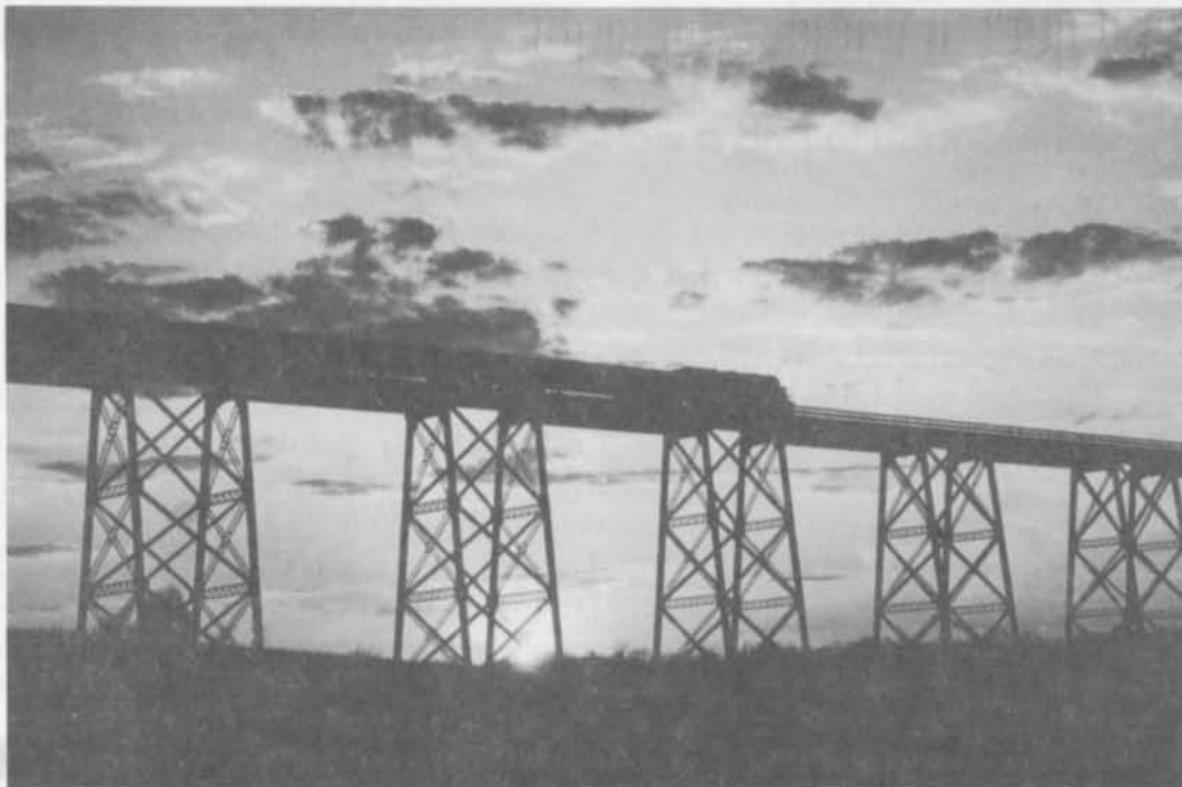
"Sundown on the Moodna Viaduct", the photograph by Pat Lecaroz took Best in Show at the Windsor Locks convention and Honorable Mention at the National Convention in Atlanta last year. The site is near Salisbury Mills, Orange County, New York.
