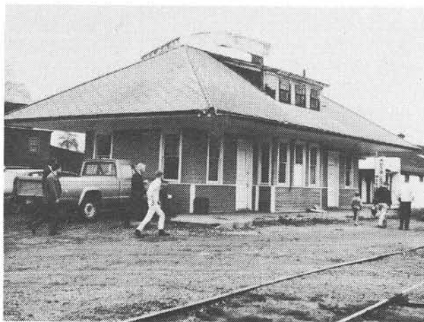
The M & E station at Morristown was a small one which could easily be modeled and used on most any home empire.
