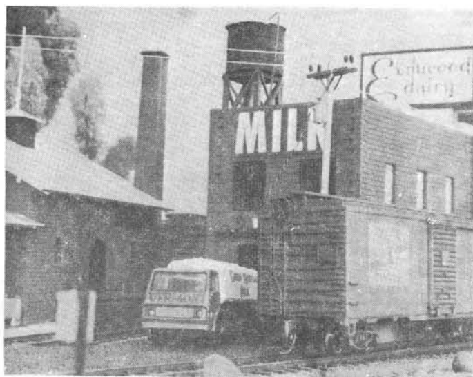
Portion of Pete Eaton's Brewery-Dairy Complex
