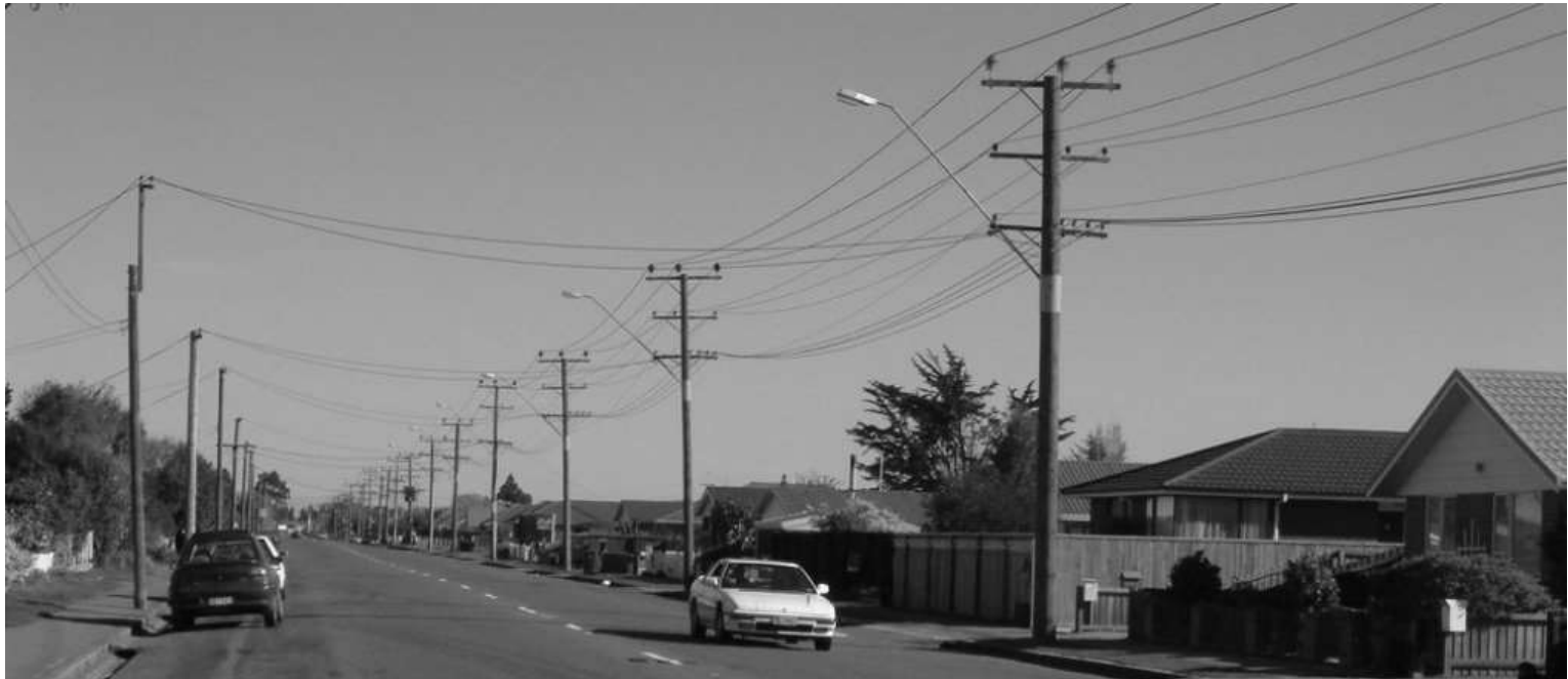
A typical street scene. Power poles on the right side of street and telephone poles on left side of street. Note extension on telephone pole. Typical power pole is 40 feet.
