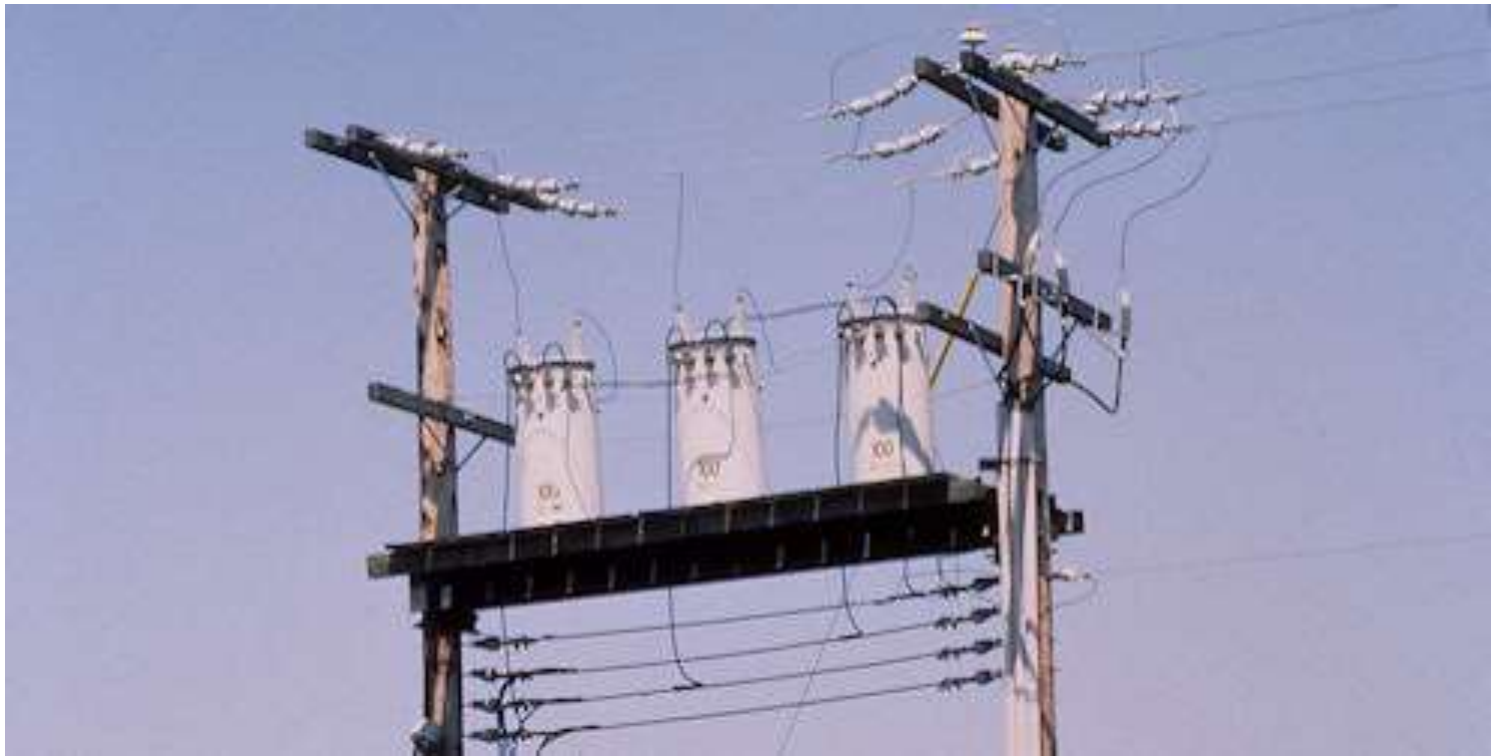
Matt style transformers mounted on a rack providing 300kva. Primary 3-phase conductors on top. Secondary service conductors on bottom. Note there are three wires for primary and four wires for secondary (277/480v-3phase-4wire)
