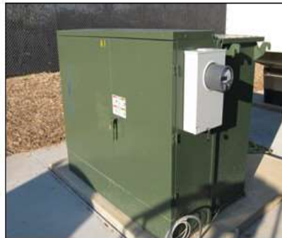
Pad mounted transformer. All wiring is underground.
